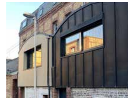
BARDAGE A JOINTS DEBOUTS Zinc
